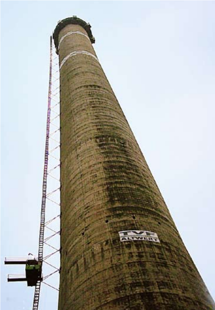
For the demolition of an industrial chimney the inner wall was systematically dismantled using a LUKAS spreader. The demolition of the chimney could not be completed using conventional methods as a blast at this location was not possible.
