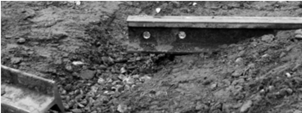
Figure 2-4. Holes Drilled in Existing Rail
