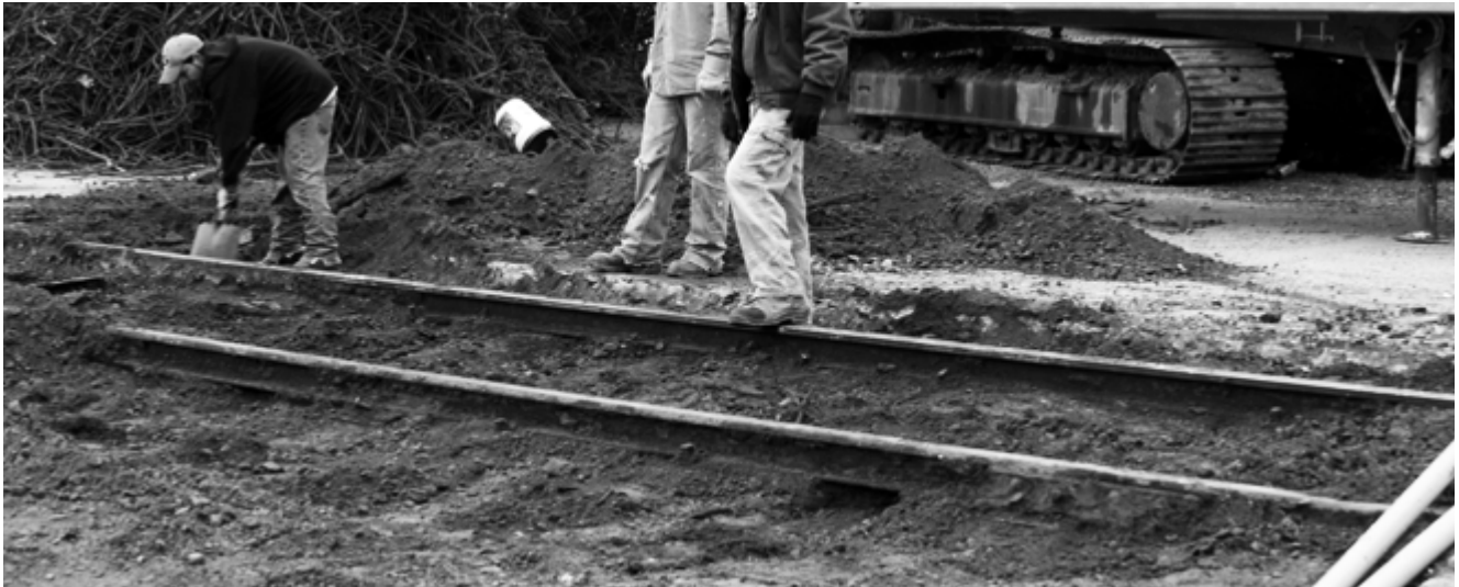
Figure 2-1. Existing Track Cleared of Ballast
