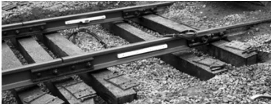
Figure 2-6. RailBoss Sections in Place
