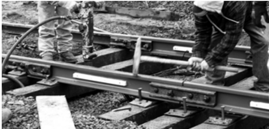
Figure 2-7. Drive Spikes Through Tie Plates
