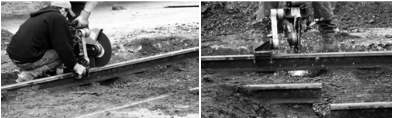
Figure 2-2. Cutting Existing Track
