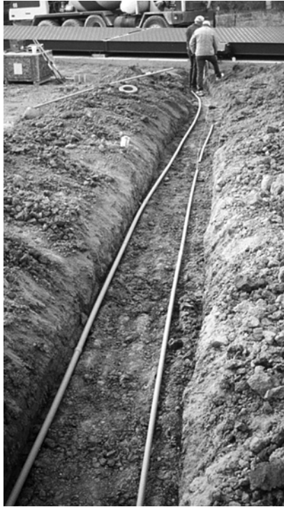
Figure 3-1. Conduit Run in Trench
