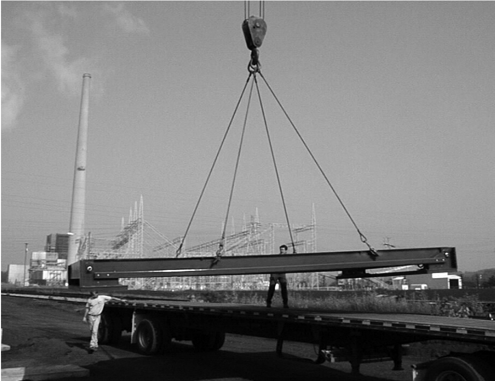
Figure 1-2. Unloading Modules From Truck
