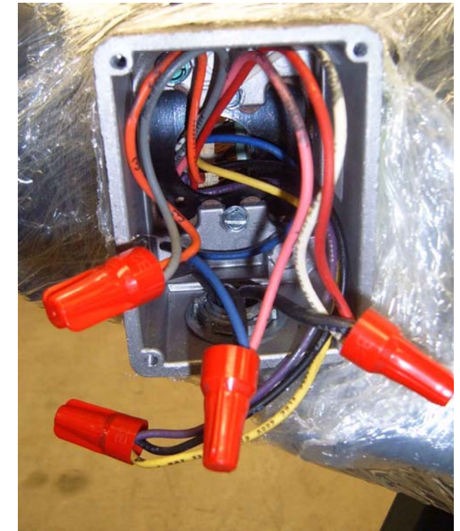
MOTOR WIRING 10 GA WIRE FROM STARTER (ITEM -90)
