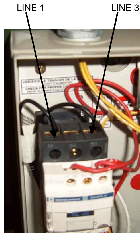
FIGURE 6-4, ELECTRICAL SYSTEM - SINGLE PHASE (Model 5000)(Optional)
