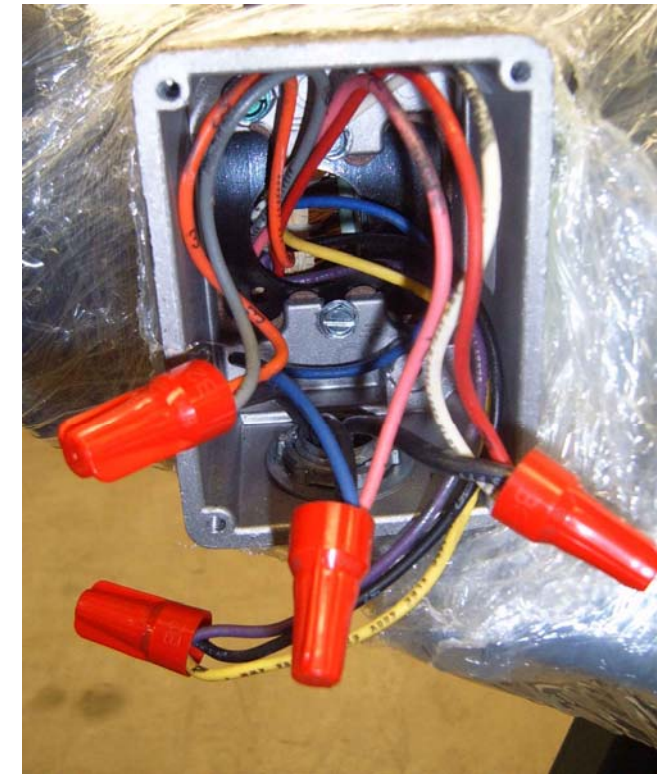
MOTOR WIRING 10 GA WIRE FROM STARTER (ITEM -80)
